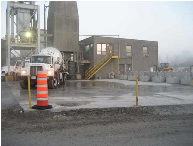
Figure 8. Completed Slab at Ready-Mixed Concrete Plant (Study 3).
