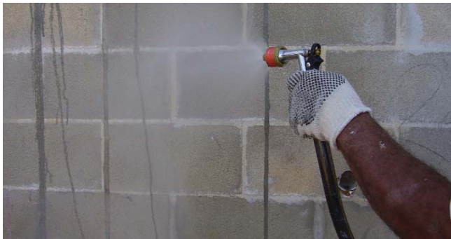
Figure 3 - Uniformly wetting the wall
